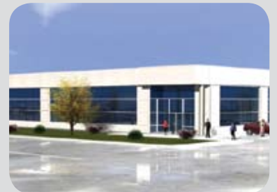
Flex Building, 6696 Financial Dr. Mississauga, ON
